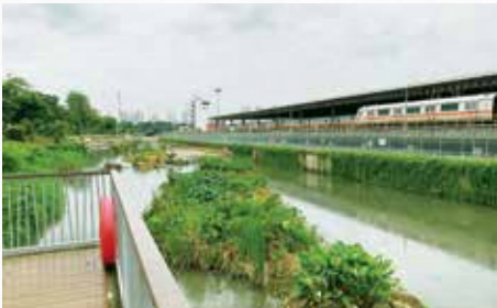
ABC Waters @ Kallang River between Bishan Road and Braddell Road have cantilevered decks along the river to allow residents to get closer to the water.
