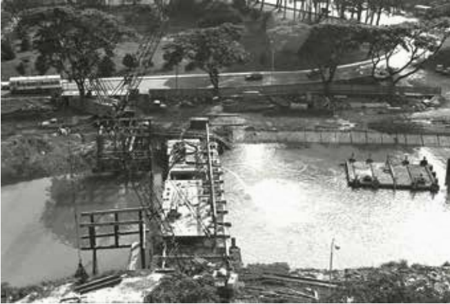
Cleaning up in progress along the river.
