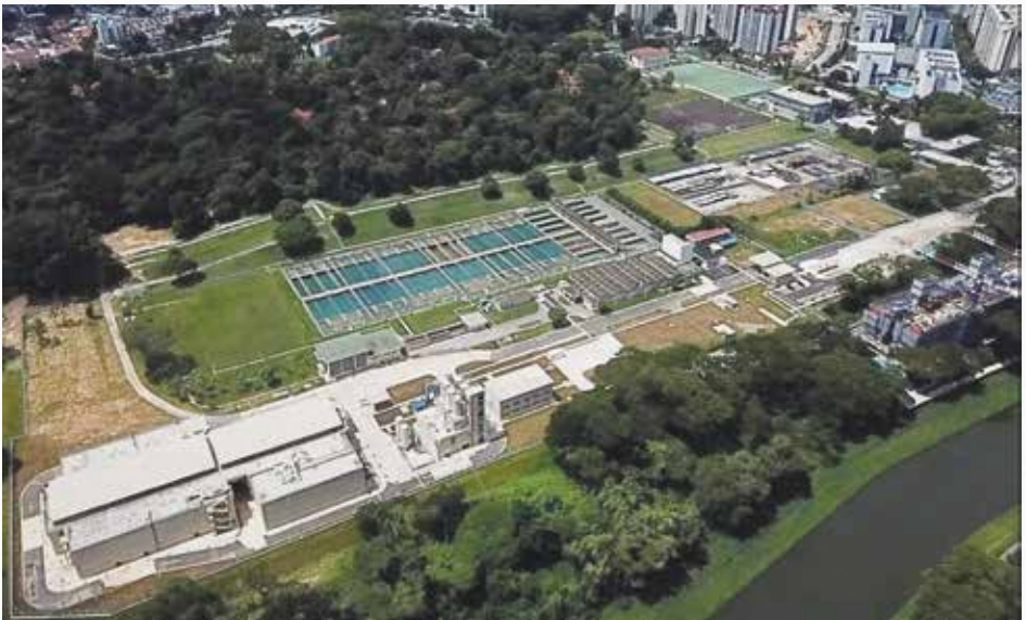
Aerial view of present day Woodleigh Waterworks.
