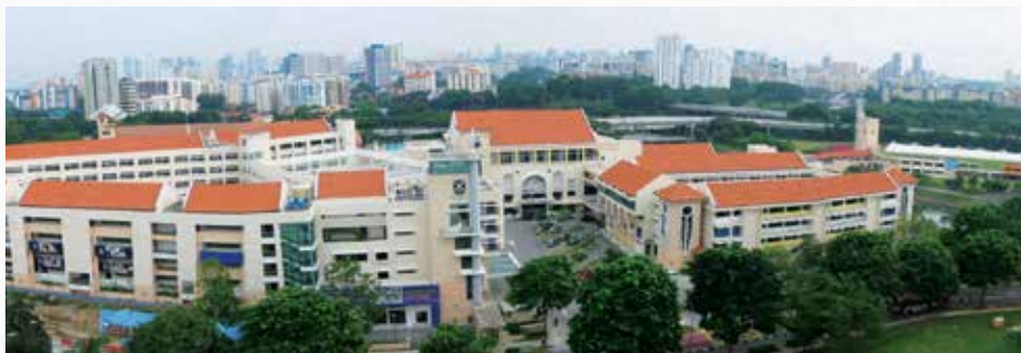
Aerial view of St Andrew's Village.
