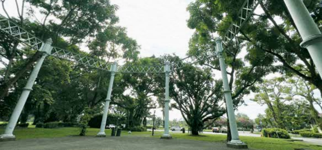
Gasholder Number 3. The steel structures were shipped from the United Kingdom.
