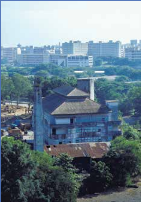
Aerial view of the Lee Rubber Factory.
