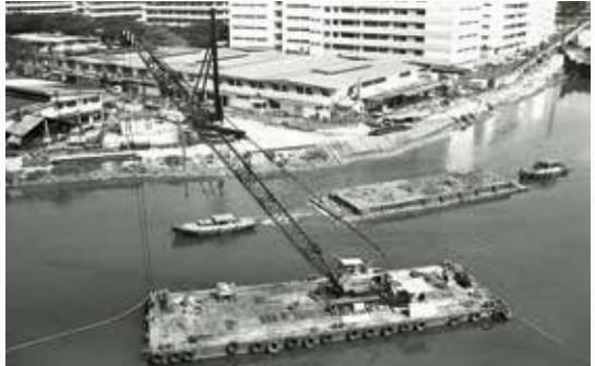
Kallang River clean-up in progress at Kallang Place.
