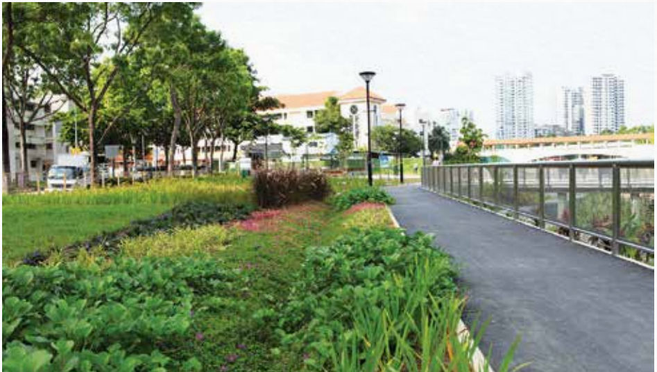
Swales at Potong Pasir with natural drainage channels and a gentle slope helps control stormwater overflow and the quality of water entering waterways.
