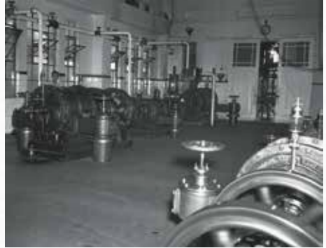
Machine room at Kallang Gasworks.
